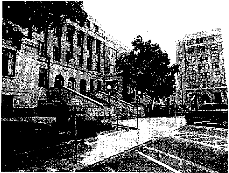
Hunt County Courthouse north entry in 2013 (ARCHITEXAS).
