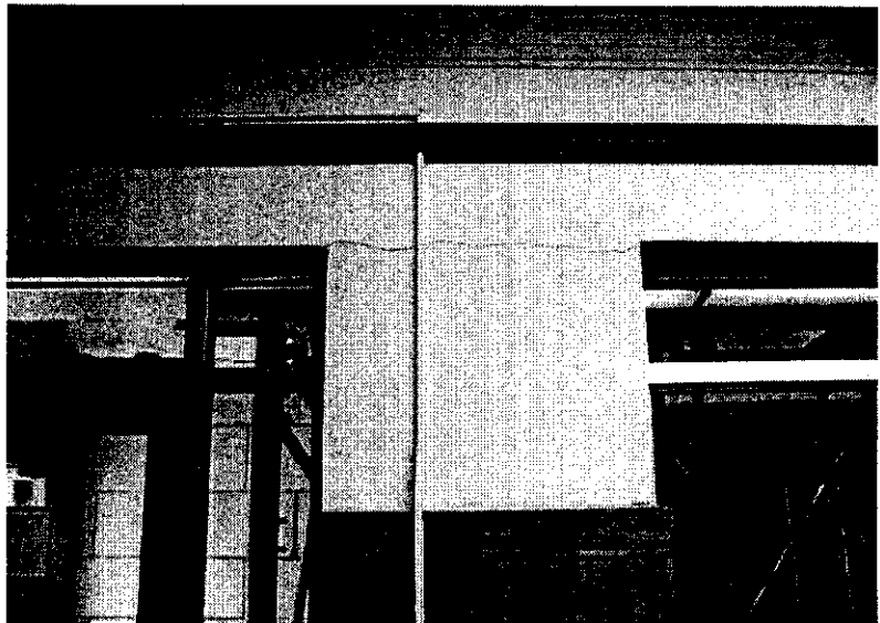
Typical cracking between doors at the entries. (Jaster-Quintanilla)
