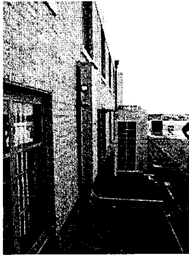
VRF system components mounted on the roof and at stair landings. (Johnson Consulting Engineers)
