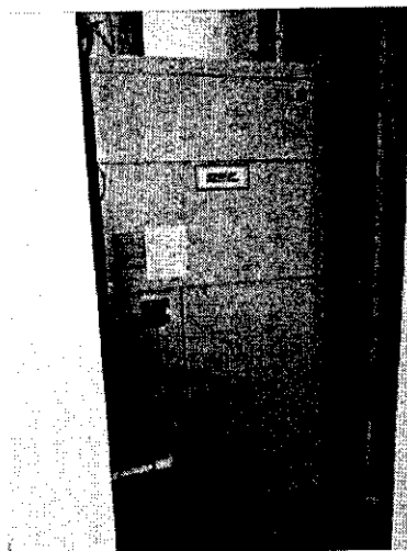
Inside units are poorly located and do not meet fire codes. (Johnson Consulting Engineers)
