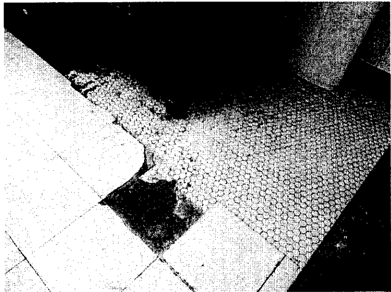
Hex tile floors in old restroom areas will require extensive rehabilitation. (Architexas)
