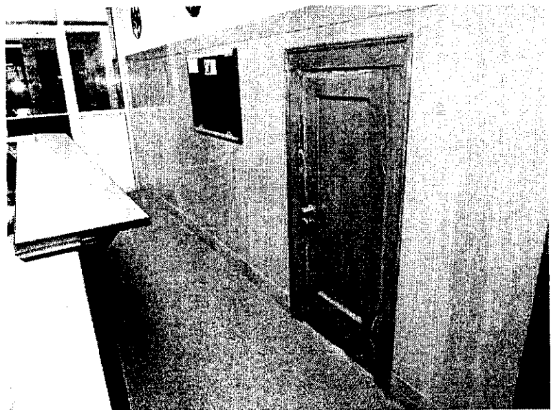
Marble wainscoting In the converted corridor at the Auditor's offices. The small door is a plumbing access hatch and is poorly sealed.(Architexas)
